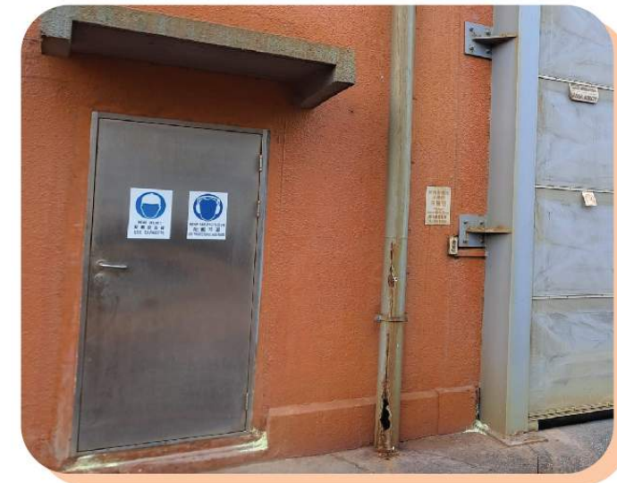
Entrance of an "Ear Protection Zone" in the power station
